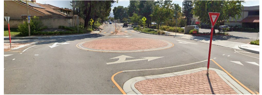
Roundabout on Duesenberg Drive and Clear Water Street
