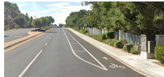
Bicycle lane with buffer on Lynn Road
