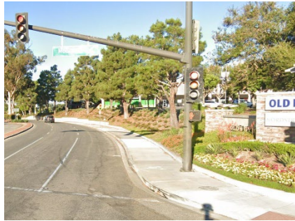
Moorpark Rd at Hillcrest Dr (Sidewalks in a commercial area)
