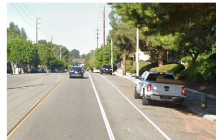
On-street edge friction (Parked vehicles and bike lanes) on E Wilbur Road
