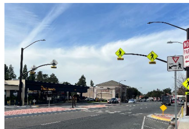
Mid-block crossing/refuge island with overhead RRFB on Thousand Oaks Boulevard
