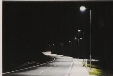
Street Lighting Alumbrado público
