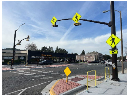
Overhead RRFBs on Thousand Oaks Boulevard
